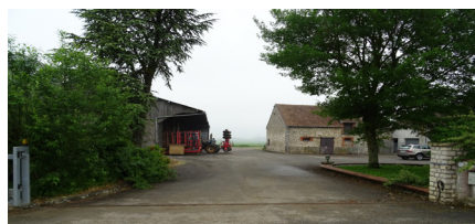
Structure agricole, Villevoques
